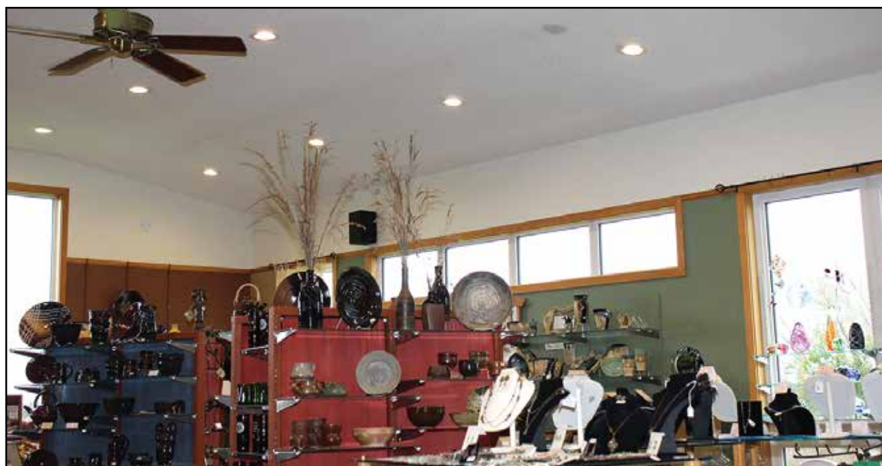
Switching to 35 LED can lights from 121 halogens cut energy use by 95% in the Gallery. The Gallery contains hand-made art from 150 artists from across the country. It's a one-stop Gallery for special occasion gifts.
