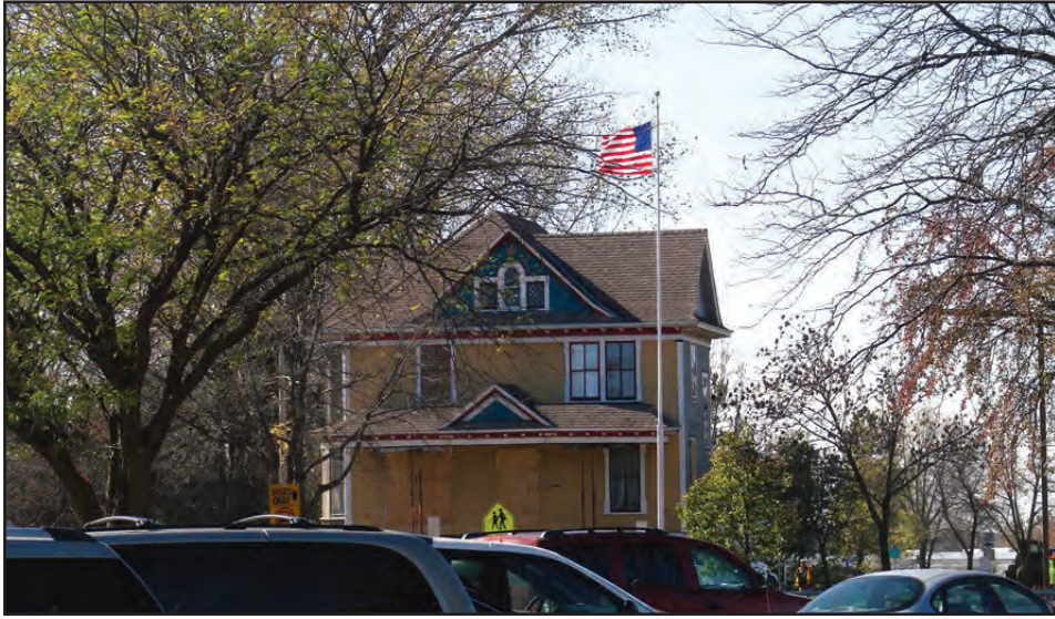
The former boarding house that stood on the lot at 201 Sibley Avenue South, Litchfield, moved through town at a snail's pace.
