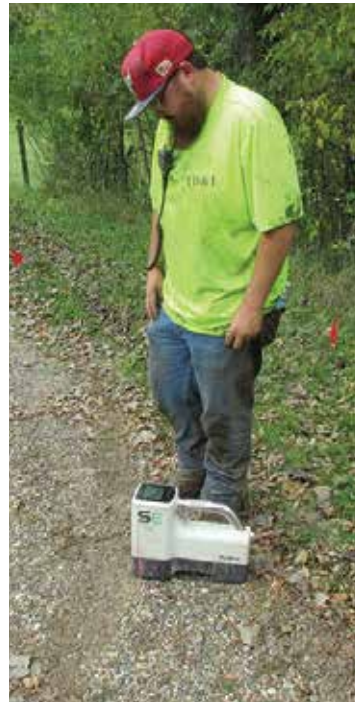
Technicians use imaging devices to check the position of the metal pipes used for boring. That sometimes means you're boring along the roadway (right photo) or even through a swampy area (photo on left). Crews are working hard to get as much boring and stringing fiber done before the ground freezes.
