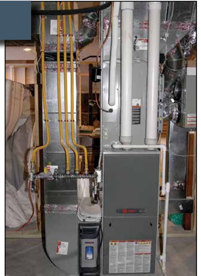
A top-of-the-line Trane air source heat pump dual fuel system switches automatically during control as well as for cost efficiency.
