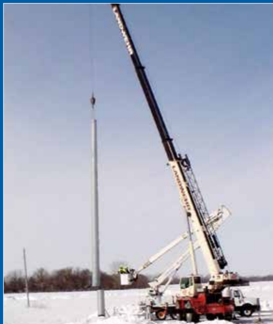
The first section of a monopole is being lifted by crane into place.
