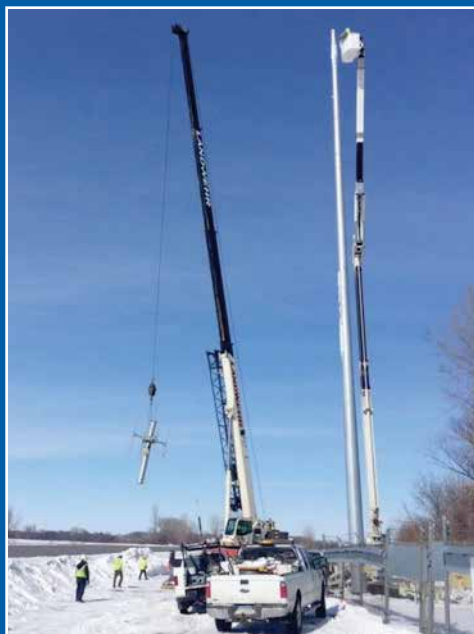
The final section—the base station—is being lifted to the top of the monopole, assisted by one of our linemen in a 120-foot bucket truck.
