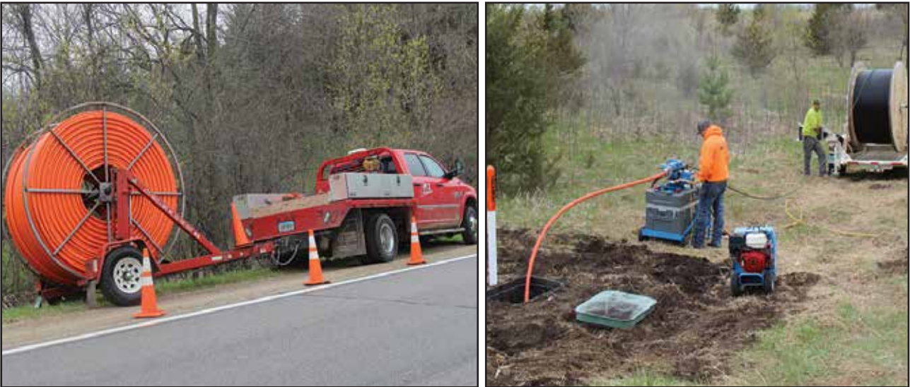
Construction continues north of Dassel near Swan Lake as crews bore holes for the orange conduit to be installed underground (left) and then blow in the black fiber cable through the conduit (right). Other crews will come behind and splice the fiber where necessary. Location #12-29-403
