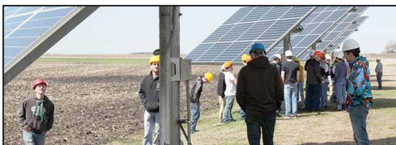
This solar installation has sensors that track the sun as well as motors that turn and tilt the solar panels to catch as much sun as possible throughout the day.
