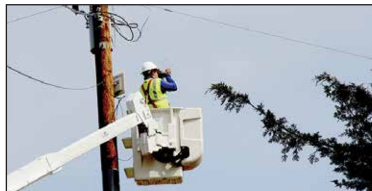
VIBRANT Broadband's Cody Schiroo does a site evaluation to see which way the receiver should point for best line of sight to the fiber-supported tower.
