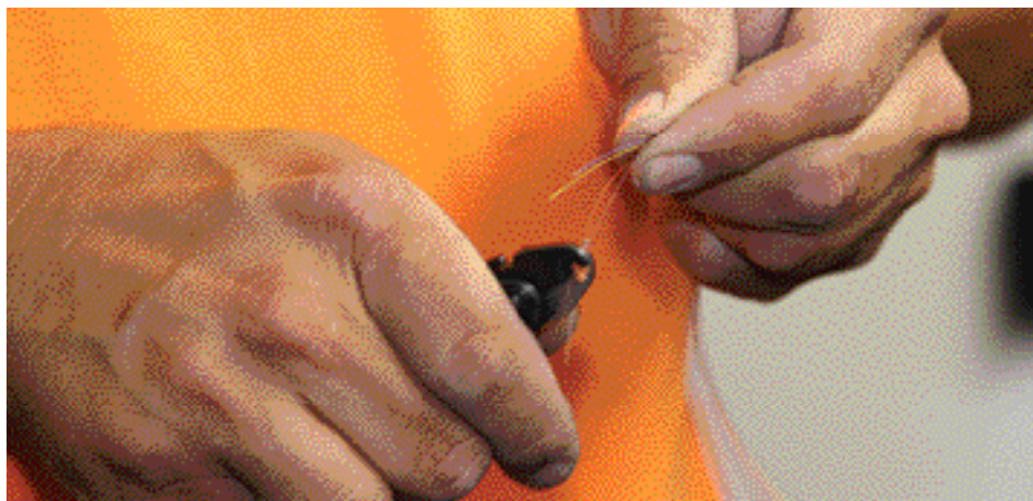
Each fiber must have the cladding removed a few inches up the fiber to prepare it for splicing.
