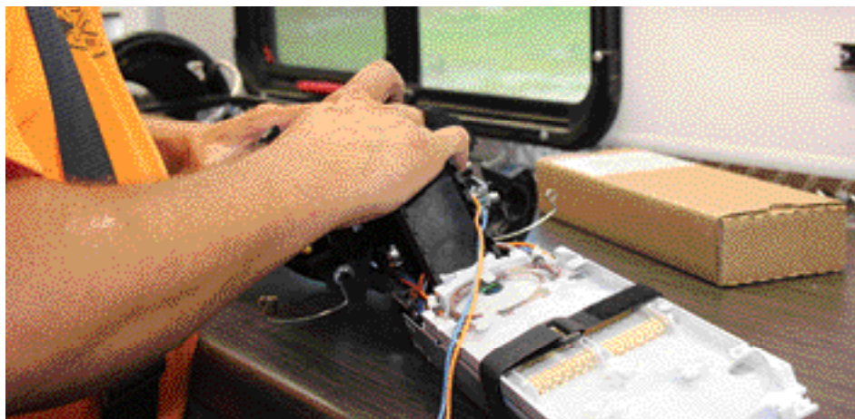
The fibers (including some extra for possible use later) are placed in a splicing tray for protection/storage.
