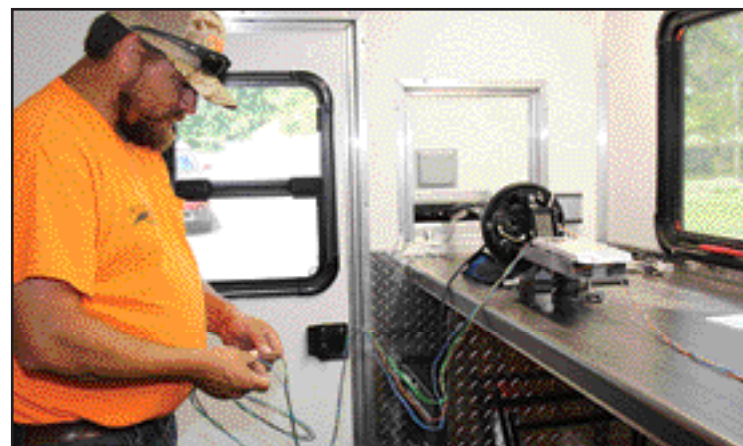
Ryan Seuss, owner of Foxtail Utilities, prepares fiber optic lines no larger than a strand of hair. These fibers will be spliced, or fused, to provide service to a homeowner.
