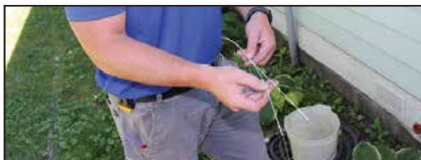
Fiber optic lines are separated and the buffering tubes must be cut away to expose the individual fiber strands that will get spliced to continue into the home. Location # 28-04-3020
